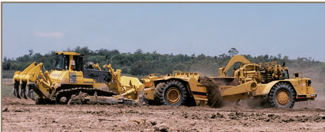
Dozer and scraper stripping top soil
