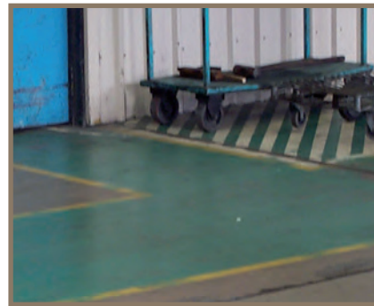
Painted floor markings
