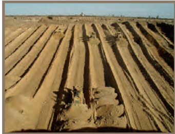
Stripping Topsoil
