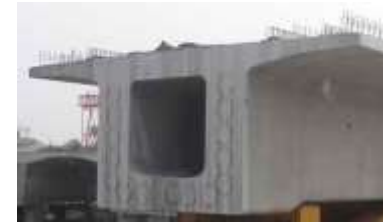
Box girders & bridge voids
