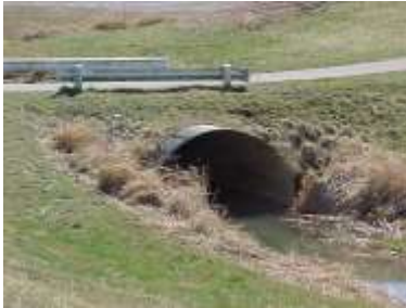
Culverts & Storm Water Systems
